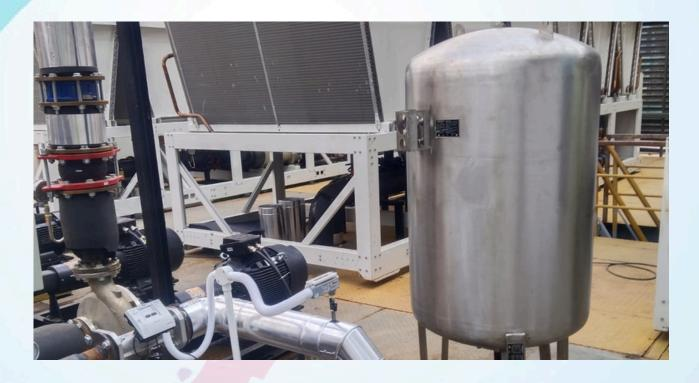
A pressure vessel is a closed container designed to hold liquids, gases, or vapors at a pressure significantly different from the ambient pressure. These vessels are widely used in various industries to store, transport, or process substances under pressure. Examples include boilers, storage tanks, and reactors.
